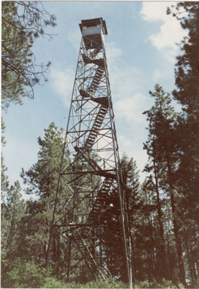
Fig. 11.2 Fire towers were often quite tall for a clear view due to the relatively gentle terrain on many forested southwestern plateaus. The 25 m tall Kanabowitz tower on the North Rim of Grand Canyon National Park was constructed in 1940 by the Civilian Conservation Corps, a Federal program that greatly expanded fire control in the Southwest (photo NAU.PH.2013.36.1.142.5, Item number 162282. Special Collections, Cline Library, Northern Arizona University)
